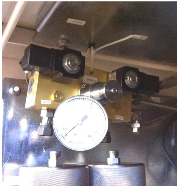
Figure 39 - Lifting the Top Manifold
